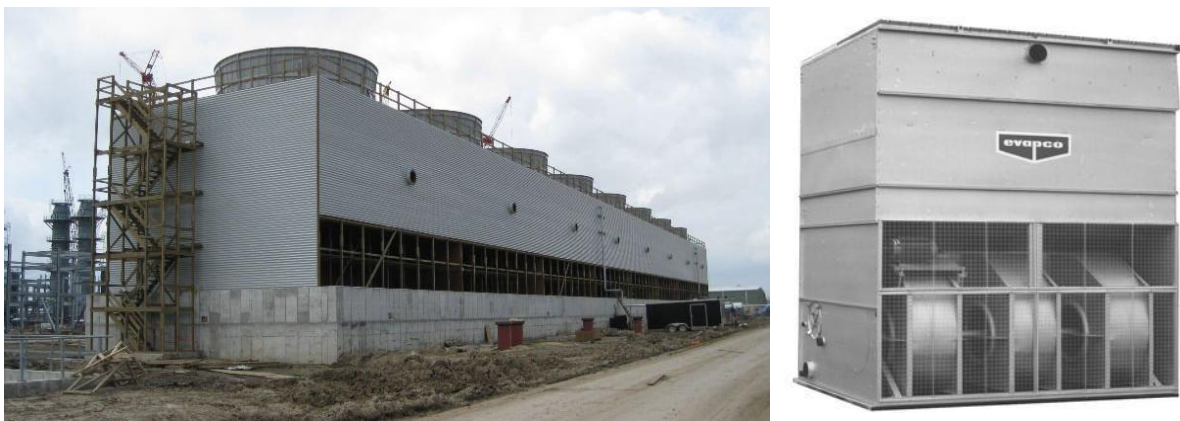
Figure 9.9 Induced draft (left) and forced draft (right) wet cooling tower example
