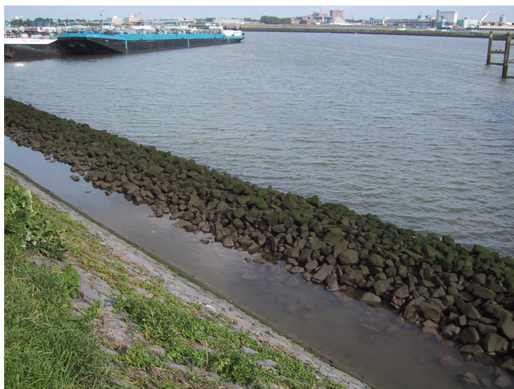
Fig. 8. View from the quay of site 2 on the shore (low tide) with the rubble bar.
