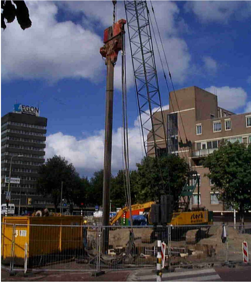
Fig. 6. Installation of temporary outer ring and permanent inner ring.
