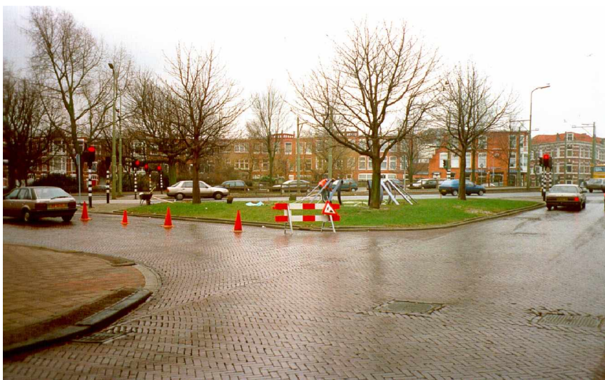
Picture S1. Site Lijnbaan/Westeinde.
