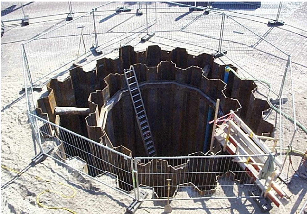
Fig. 7. Excavation inner and outer ring.
