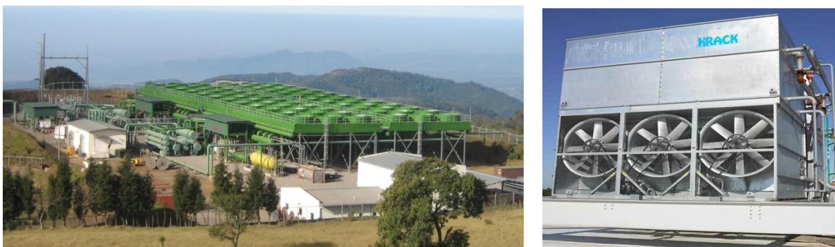
Figure 9.10 Induced draft (left) and forced draft (right) air cooling examples
